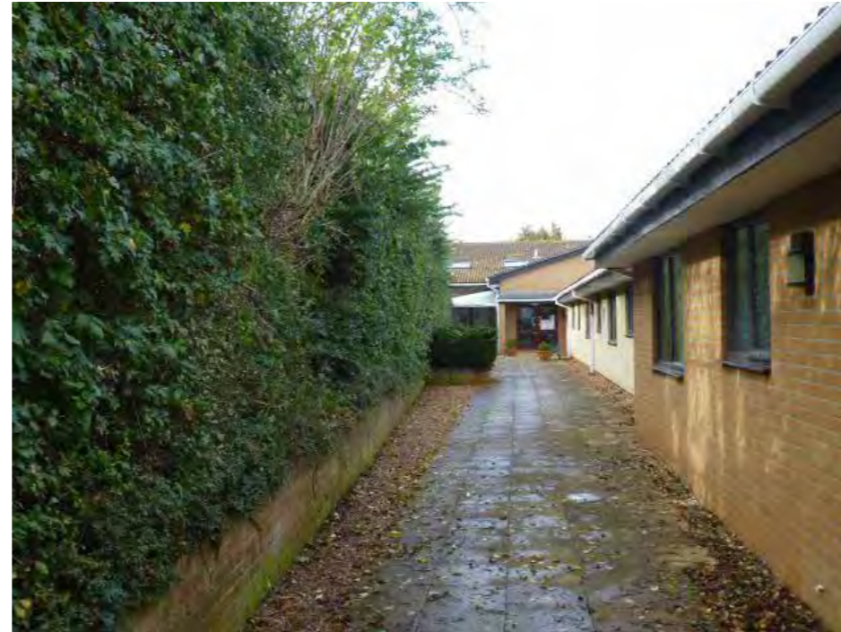
5. Proximity of Parkside Ward South Elevation
